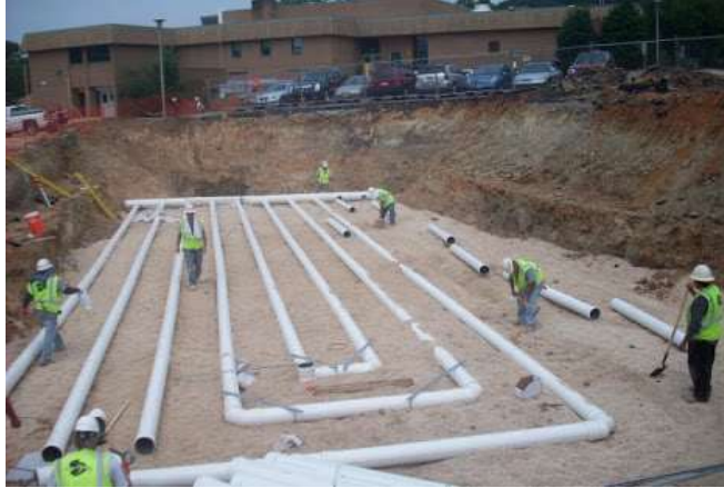
Fig.3 Installation of Earth Tube
